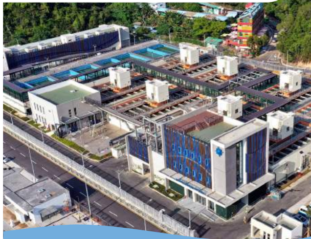
澳门石排湾净水厂 Macao Seac Pai Van drinking water treatment plant
