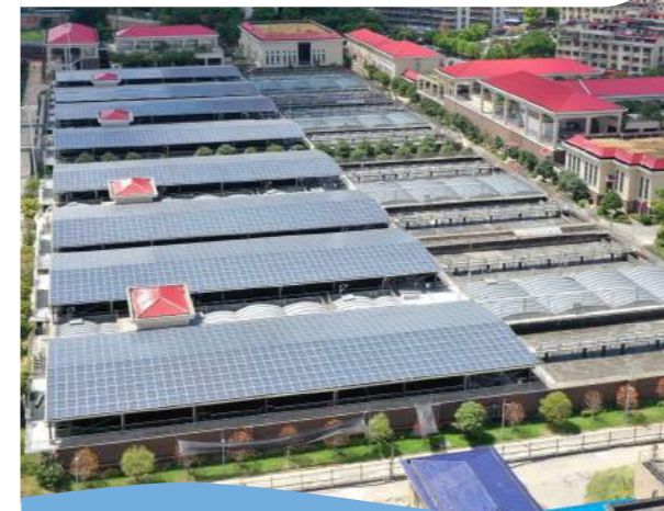
长沙市开福污水处理厂 Changsha Kaifu wastewater treatment plant
