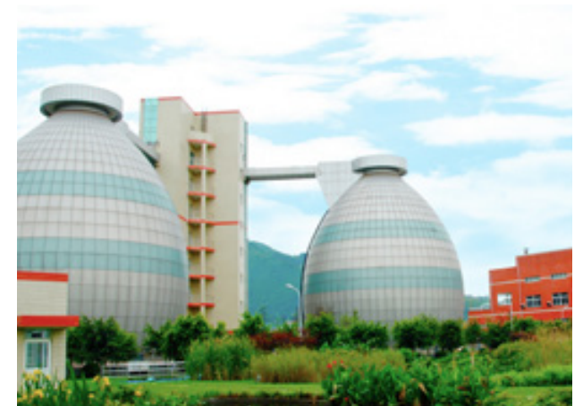
▲ Chongqing Tangjiatuo wastewater treatment plant was recognised by the industry as a benchmark for sophisticated operation and management of wastewater treatment.
