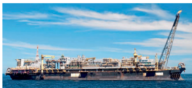
* FPSO = Floating, production, storage and offloading
