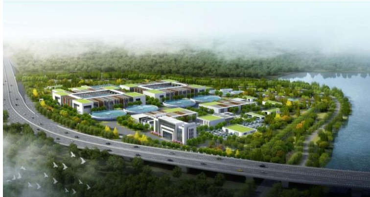
At RMB 7.25 million, the Changshu Chengdong wastewater plant has a daily capacity of 120,000 m 3 /day
