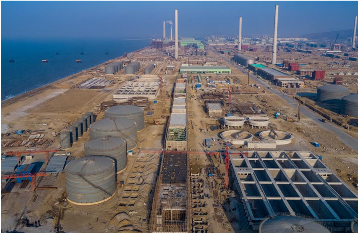
Refinery WWTP in Construction for the 20 million tons/year Refining-chemical Project
